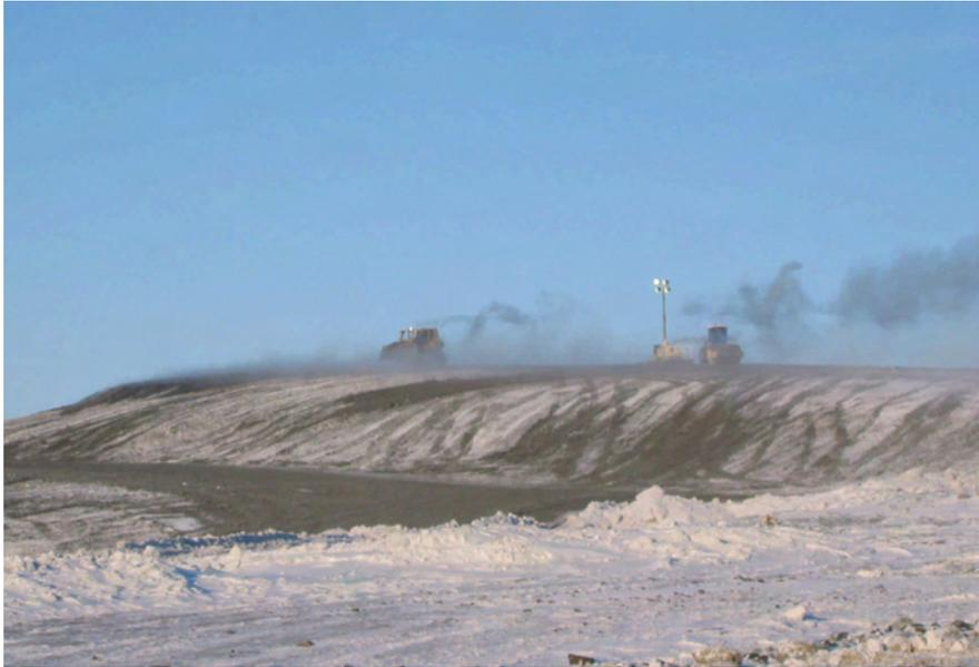
**Figure 6-5. Tailings being spread and compacted on stack**
