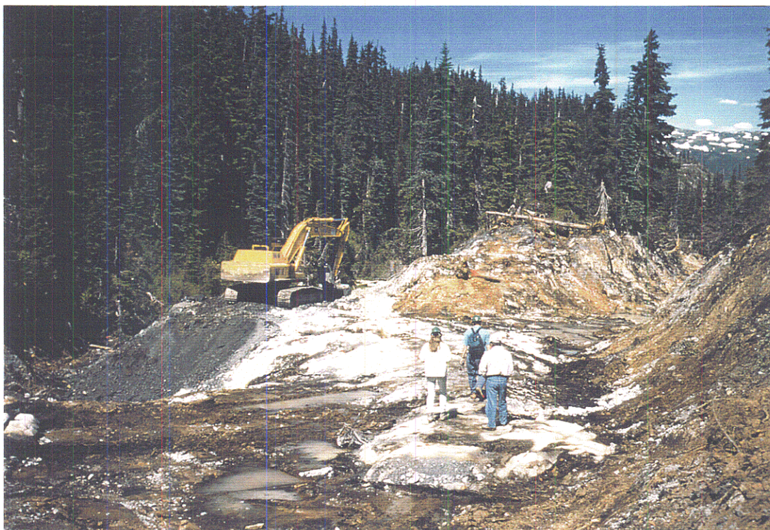
Photo 9. After dump disassembly, looking northeast with bedrock knob in left middleground; small valley to left of knob returned to pre-dump contours (see Photo 1).
