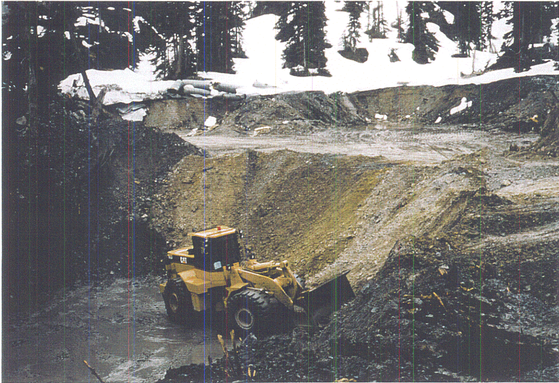
Photo 3. During dump disassembly; dump disassembled in lifts (layers); note orange-brown oxidation.
