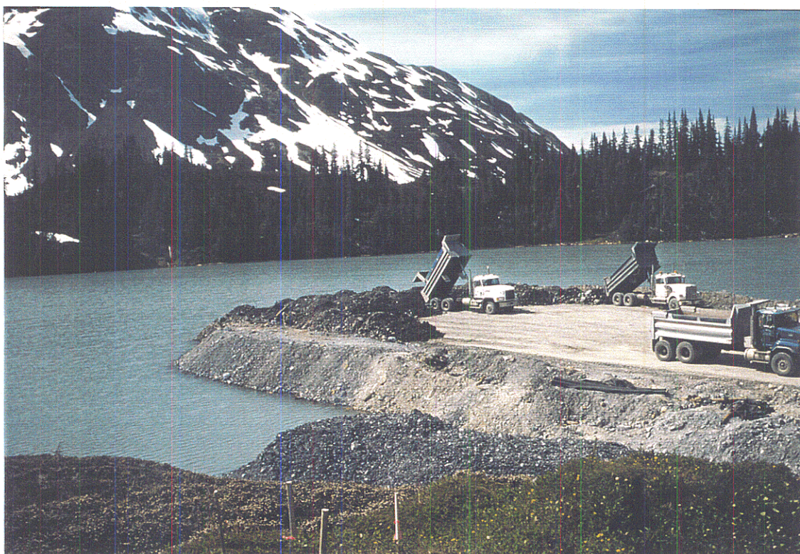
Photo 10. During dump disassembly; placement of excavated waste rock in nearby lake.
