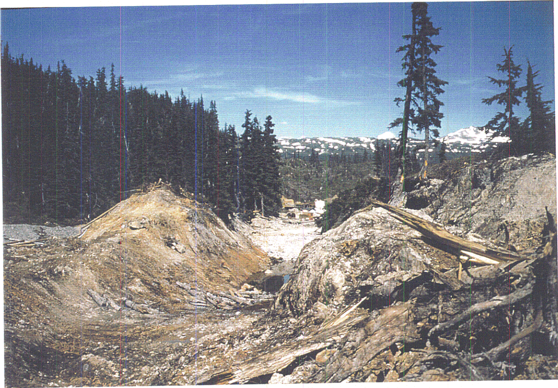
Photo 7. During dump disassembly, looking northeast with bedrock knob in right background.
