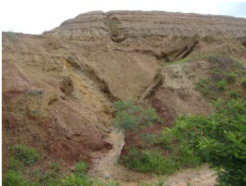
Figure 1 Thinly covered vegetation at New Union Gold Mine tailings showing water erosion
