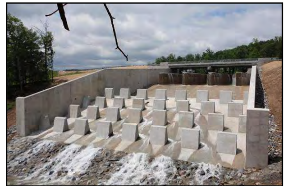
Figure 2 Spillway and Energy Dissipators
