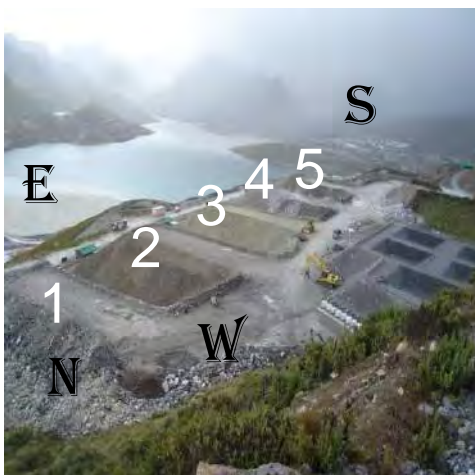
Figure 1 Photo of the five experimental waste rock piles
