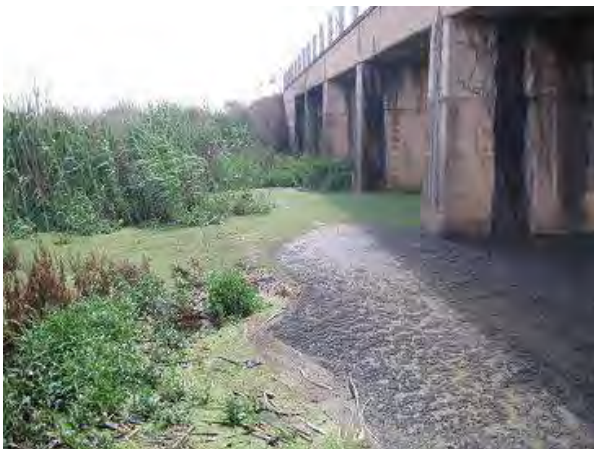
Figure 8 Raw sewage discharged into the Blesbokspruit
