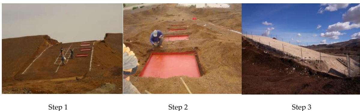
Figure 2 Photos illustrating the field inclined SR cover construction steps
