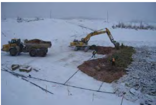
Figure 1 Construction of the field-based BCR showing the perforated feed pipes, organics (brown) and rock (right-hand side) layers.
