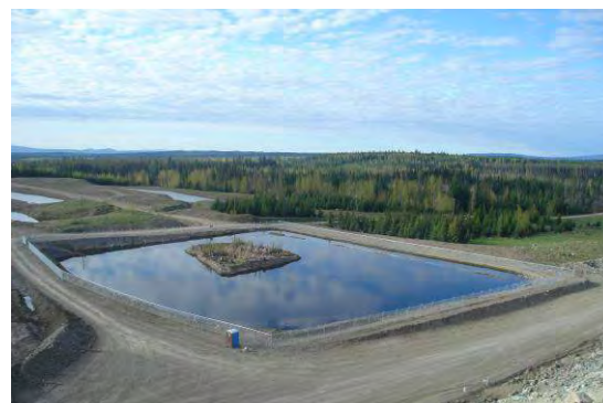
Figure 2 View of the completed BCR looking down from the top of the tailings storage facility.
