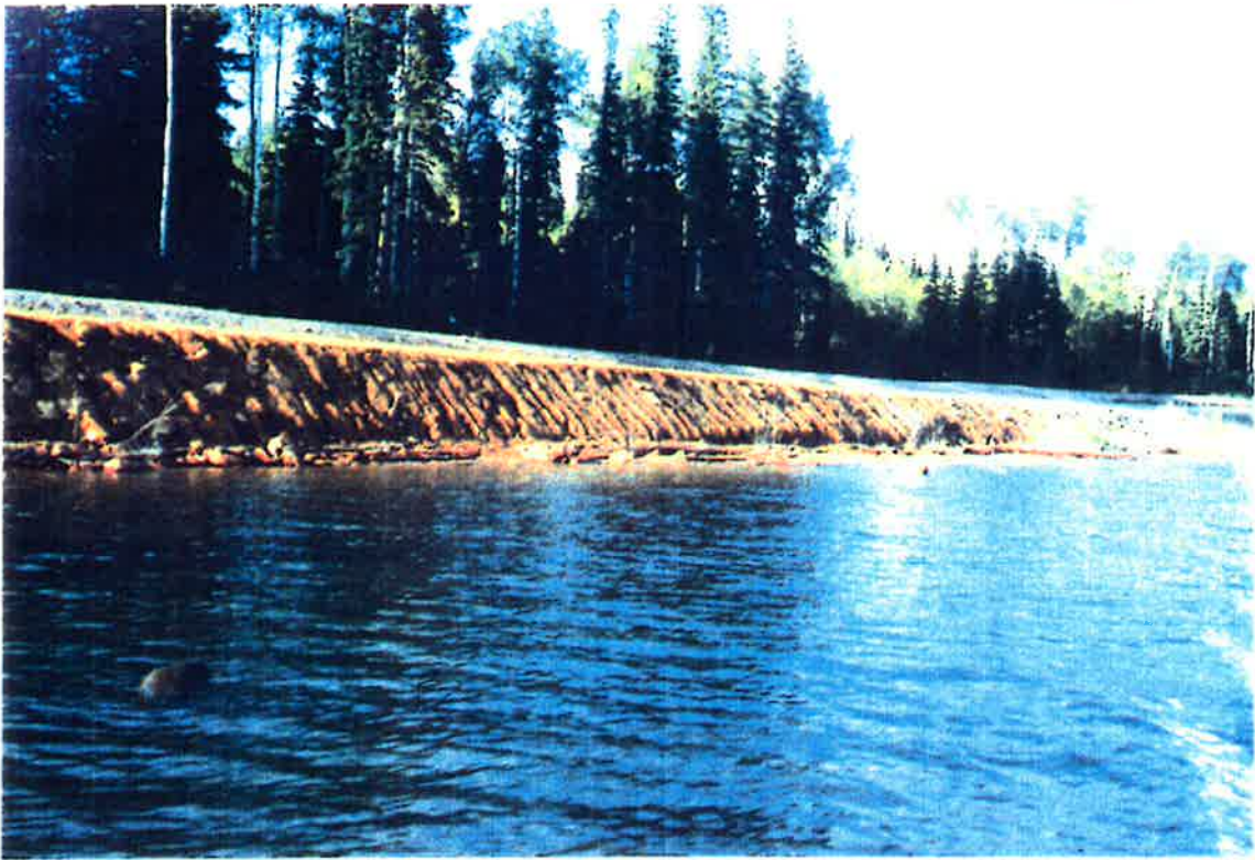
Plate 3-11: Road located adjacent to Anderson Lake built from mine tailings (Zone C).
