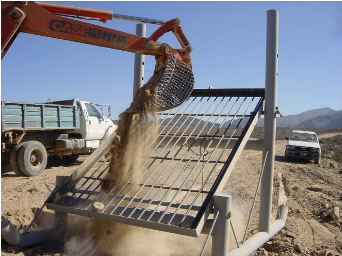
Figure 3.2 Large-scale field screen (grizzly) used to remove material greater than 100 mm.
