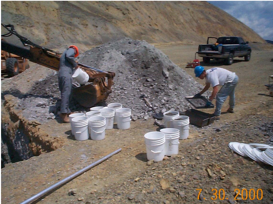
Figure 2.3 Sampling borrow pit material.
