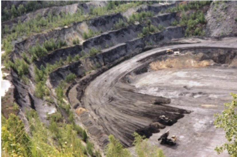
**Figure 11-11 Advanced Stage of Pit Backfilling (2002, M. Paul) [16]**
