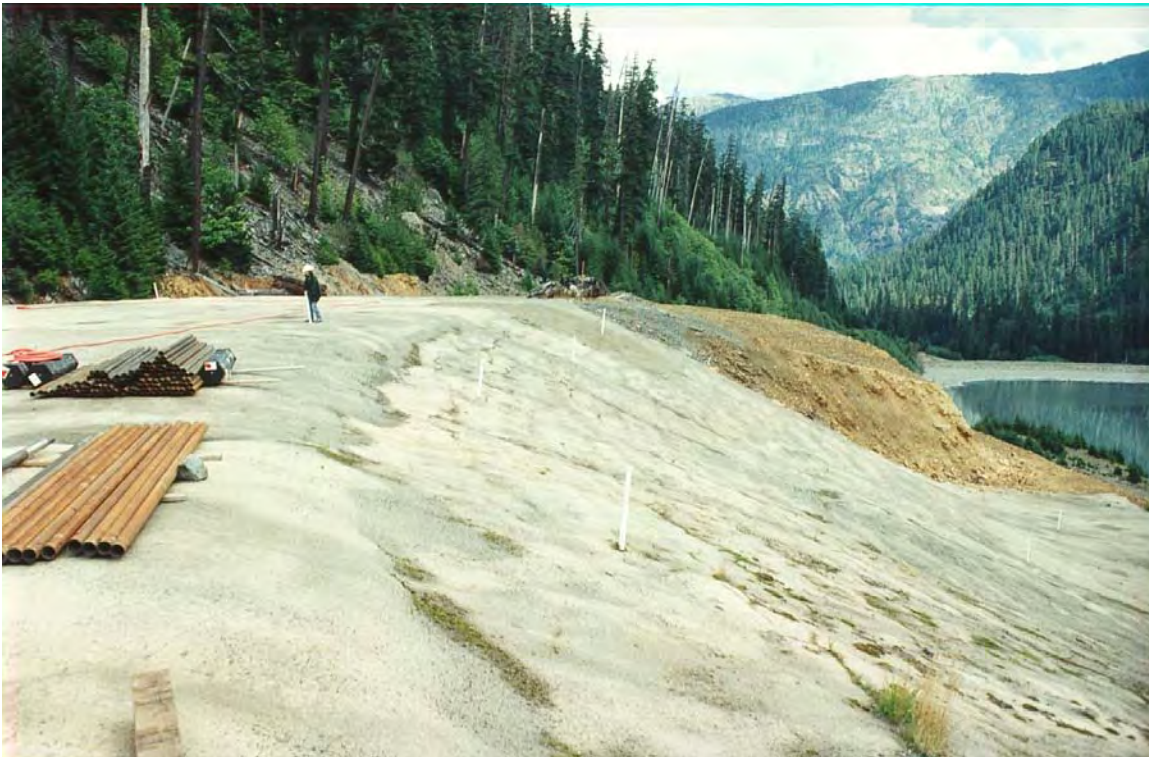
Fig. 3.1. View of Myra Falls Shotcrete Cover showing sharp change in slope (Photo by M.D. Haug).
