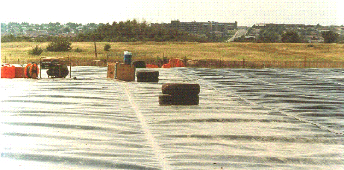
Fig. 4.8 – Construction of U of S Chemical Landfill Cover (Photo by M. D. Haug).
