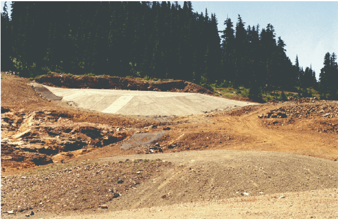
Fig. 3.2. View of Mount Washington Shotcrete Test Cover (Photo by M. D. Haug).
