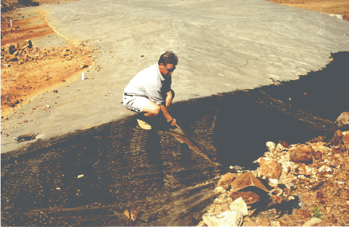
Fig. 4.13 – Asphalt emulsion/ geotextile waterproof membrane (Photo by M. D. Haug).
