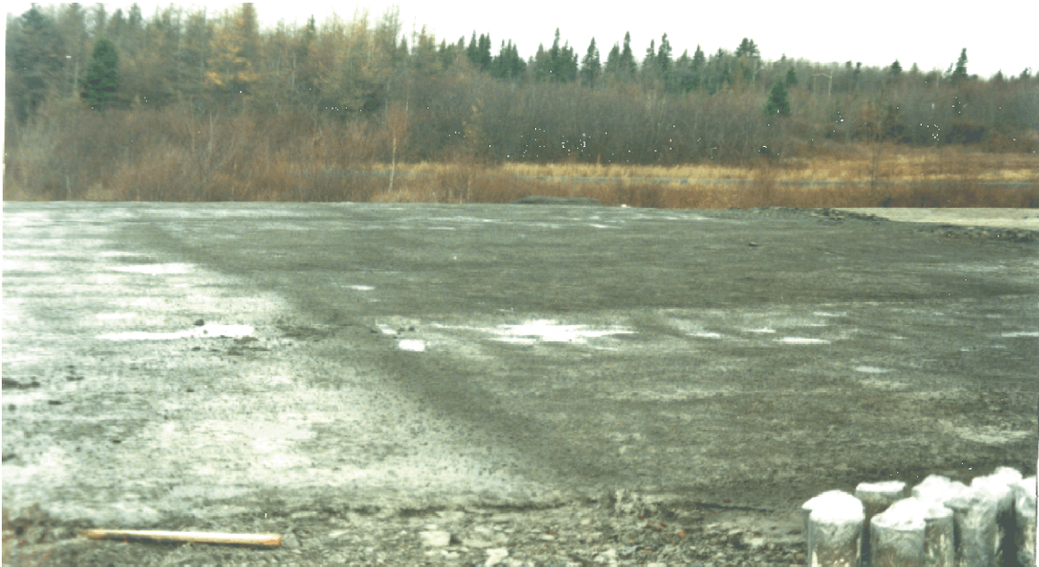
Fig. 3.3 – Halifax Shotcrete Test Covers (Photo by M. D. Haug).
