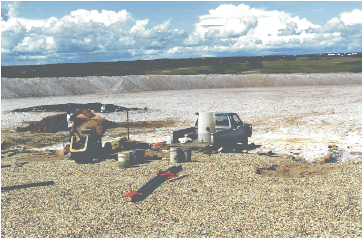
Fig. 5.2 – Repair Work on the Soil Bentonite Test Cover at the Patience Lake Potash Mine in Saskatchewan (Photo by M. D. Haug).
