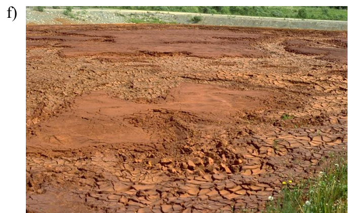
Plate 22. Sustainable Vegetation and Acidic Drainage – Common Misconception of the 1970s a) Simple Vegetation Cover b) Oxidized Surface Layer of Tailings below Cover c) Toe of Tailings Dam d) Acidic Drainage e) Treatment Plant f) Lime Treatment Sludge Pond
