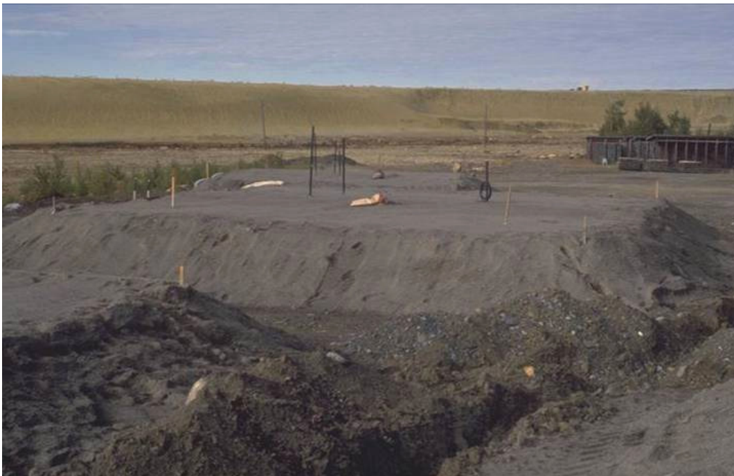
Plate 8. Field Test Cell – Dry Cover.
