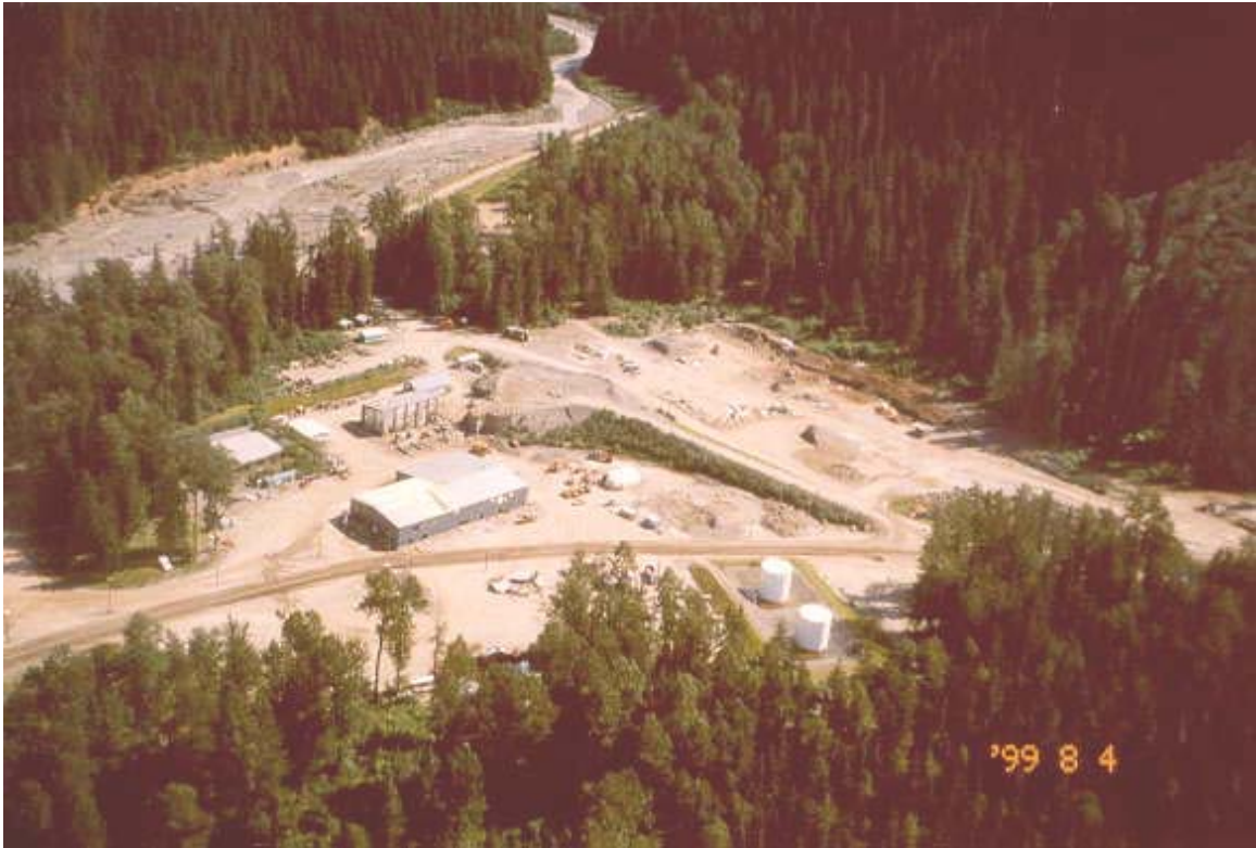
Photo 1. Plant Site and Camp with Bronson Creek in the Background
