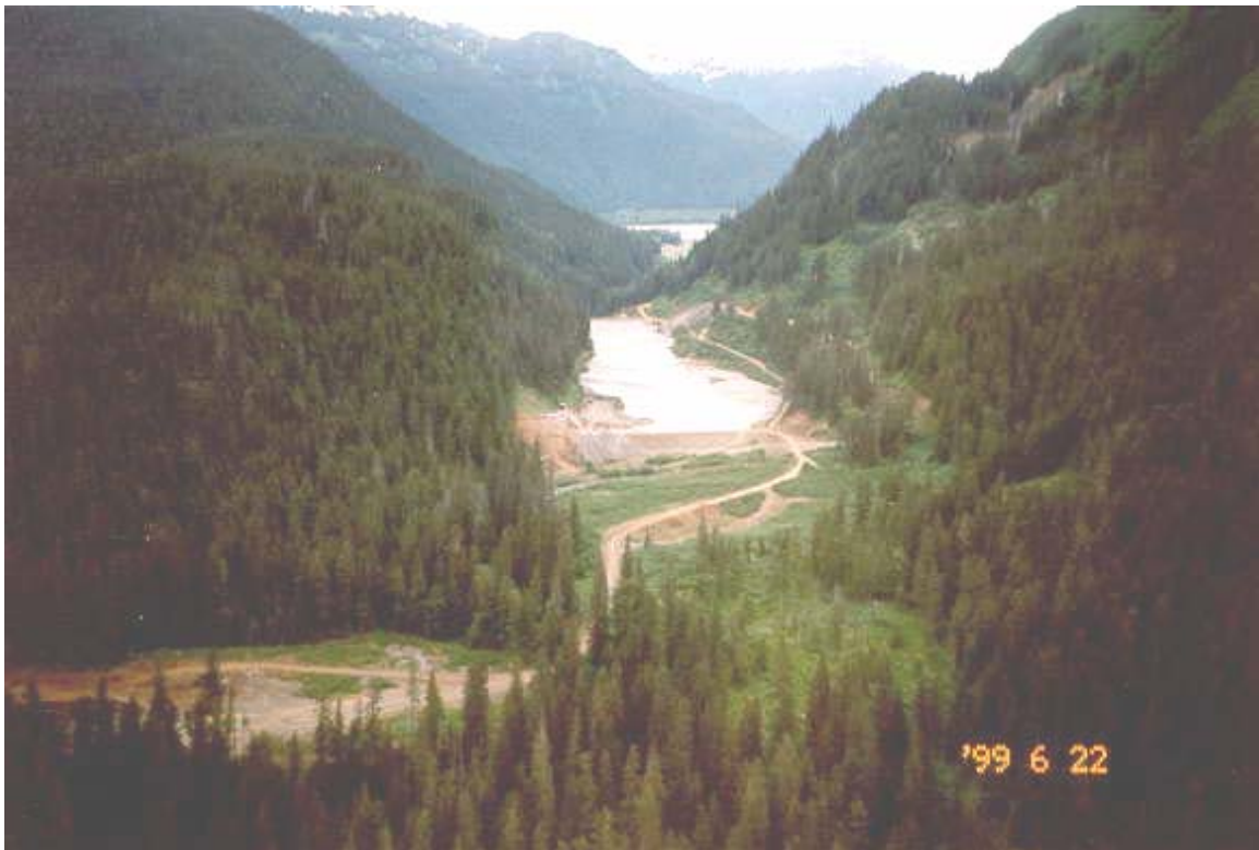
Photo 2. Tailings Impoundment with Main Underground up the Slope to the Right
