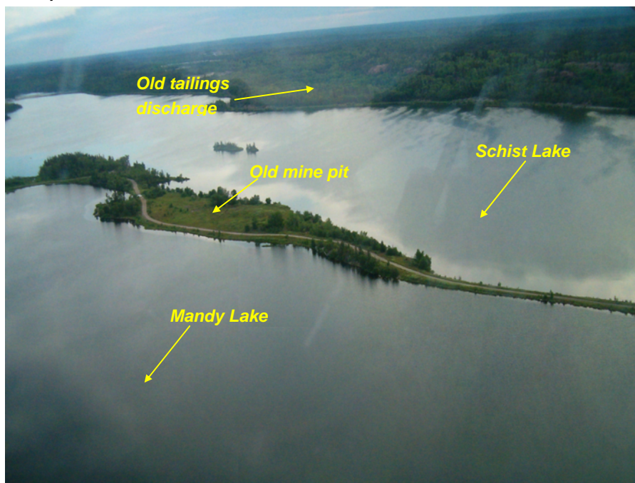
Photo 6-3 - Mandy Lake Mine After Reclamation in the Early 90's (Looking Northeast) (Source: HBMS)
