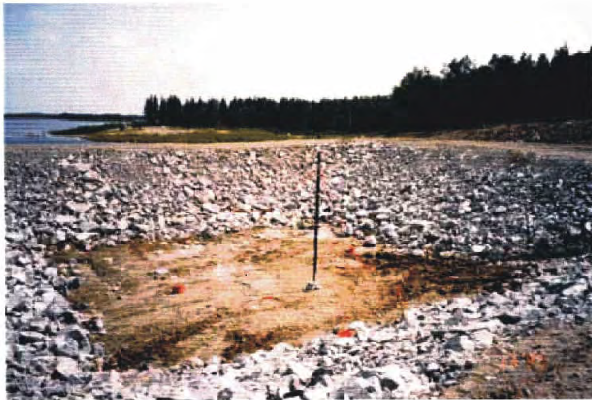
Picture 2: Cell #1 before filling.
