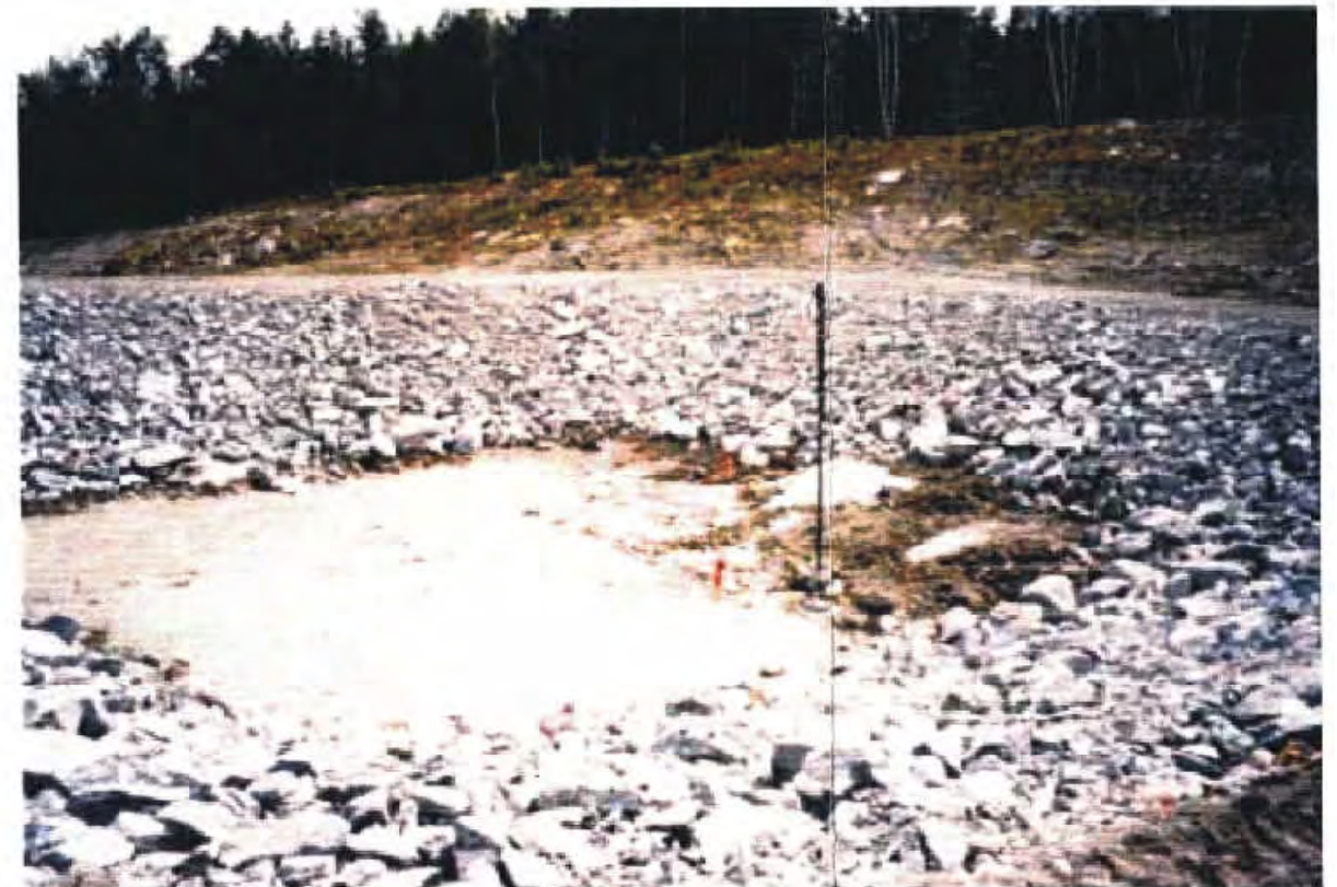
Picture 3: Cell # 2 before filling.
