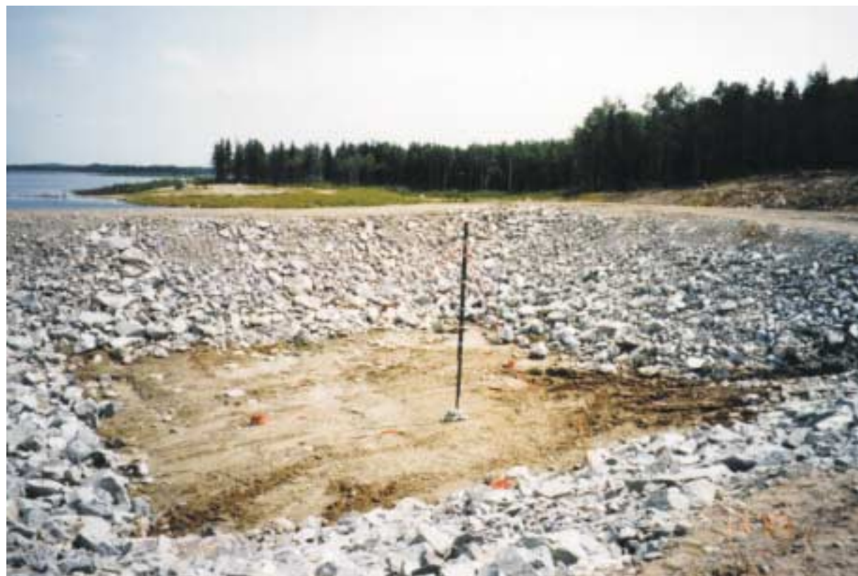
Picture 2: Cell #1 before filling.
