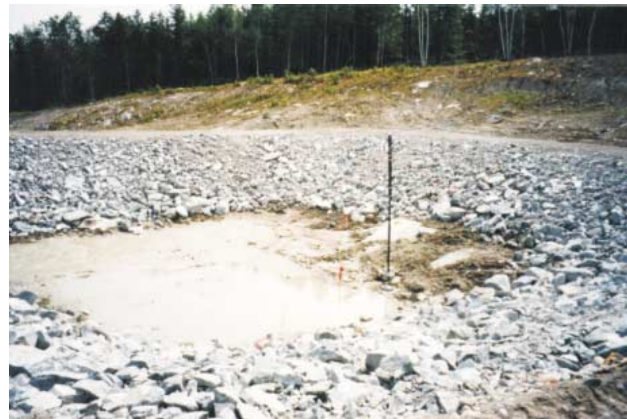
Picture 3: Cell # 2 before filling.
