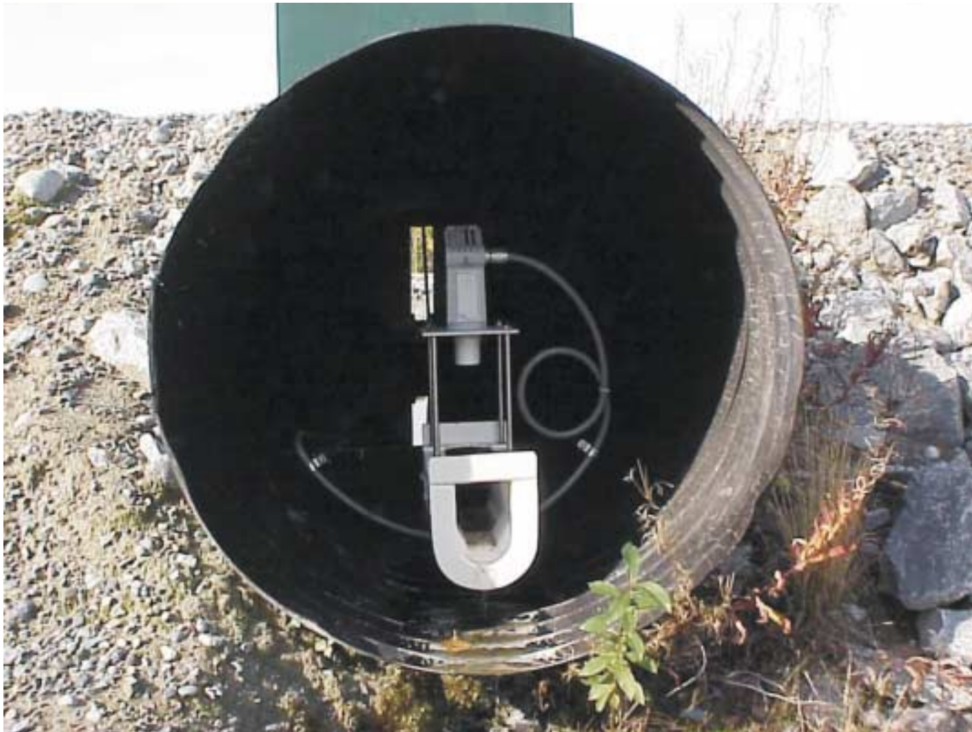
Picture 8: Outflow of the spillway and flowmeter.
