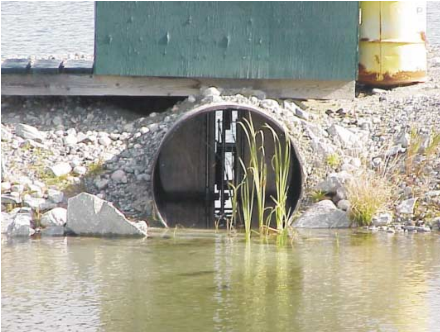
Picture 7: Intake of the spillway pipe.
