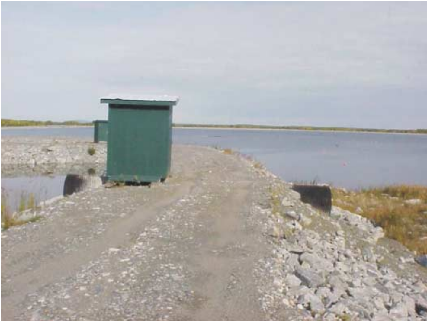
Picture 5: Monitoring cabin over the instrumented spillway.
