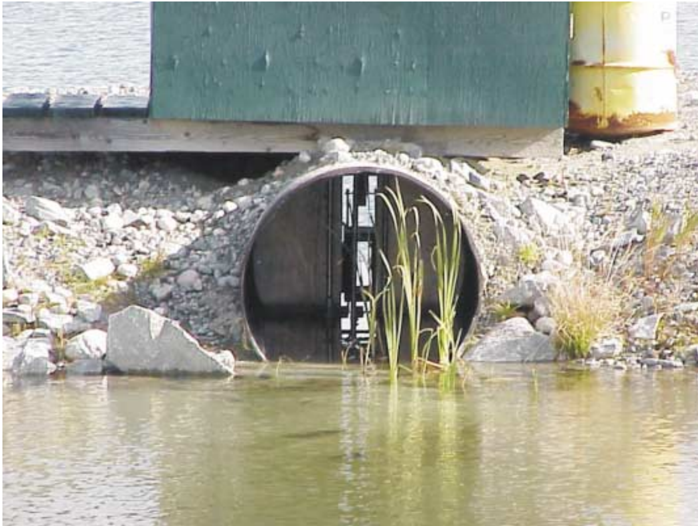
Picture 7: Intake of the spillway pipe.
