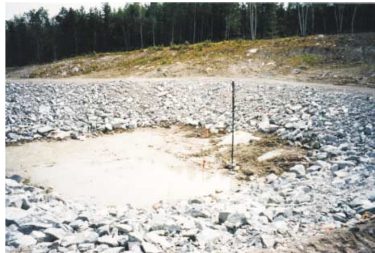
Picture 3: Cell # 2 before filling.
