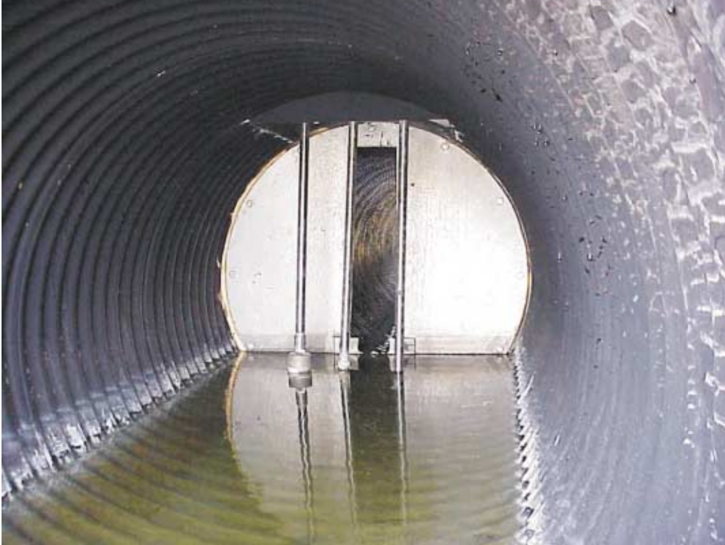
Picture 6: pH meter within the spillway pipe.
