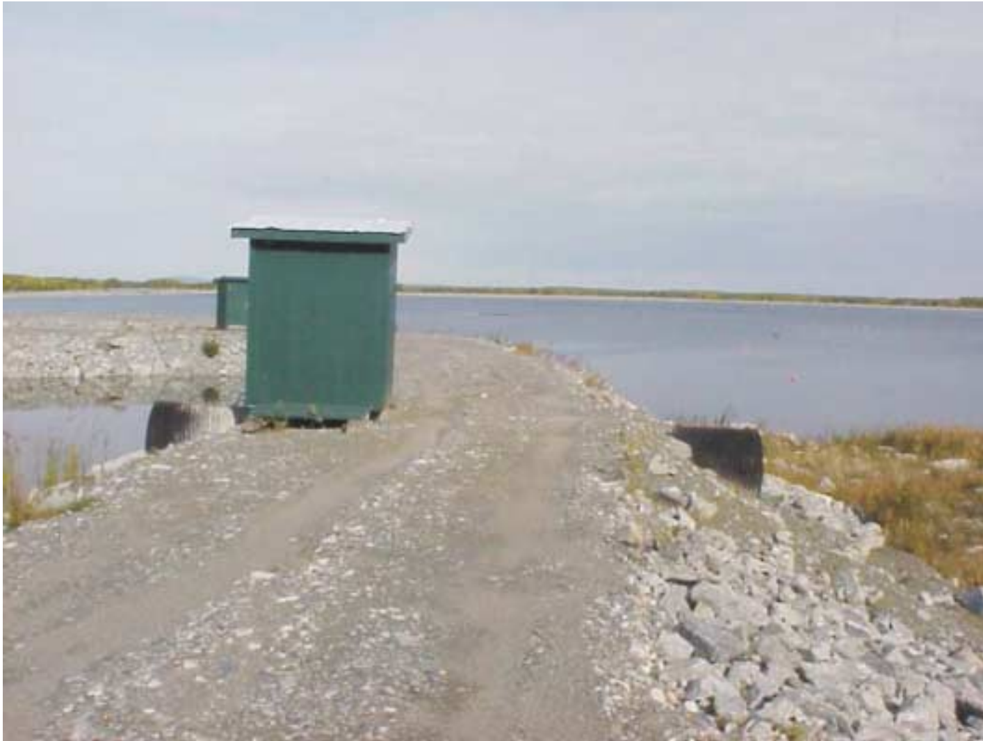
Picture 5: Monitoring cabin over the instrumented spillway.
