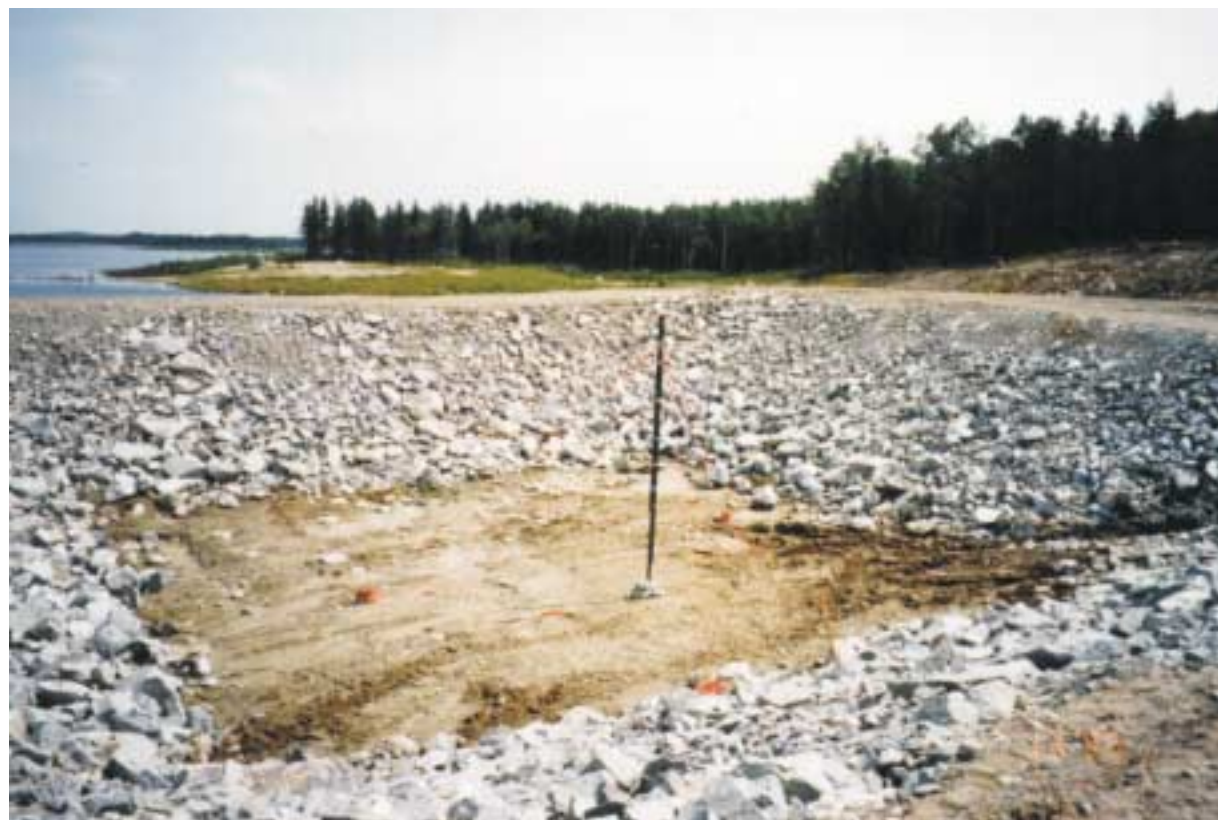
Picture 2: Cell #1 before filling.
