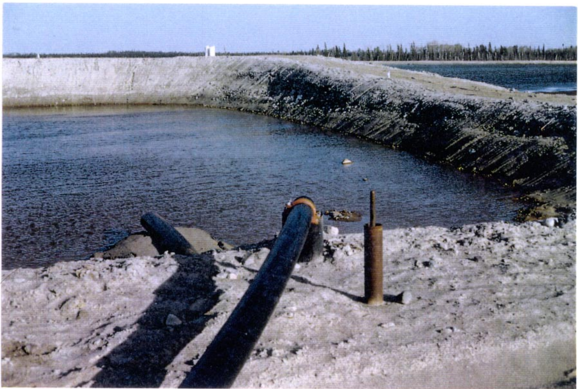
Figure 3-3: View of test cell with pipeline in place to supply fresh water from Sturgeon Lake. Photograph taken on May 20, 1992 before the water was pumped out (July 7-9, 1992).
