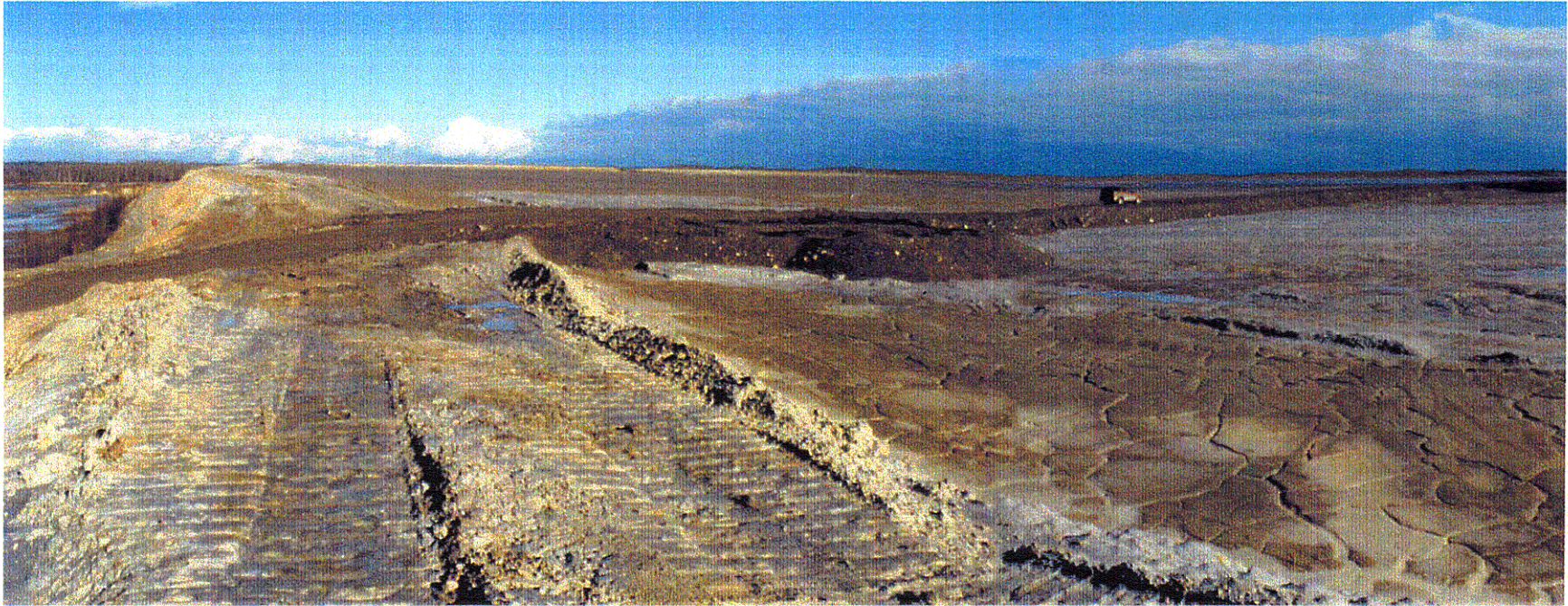
Photograph 5: Stack surface before construction (fall 1995)
