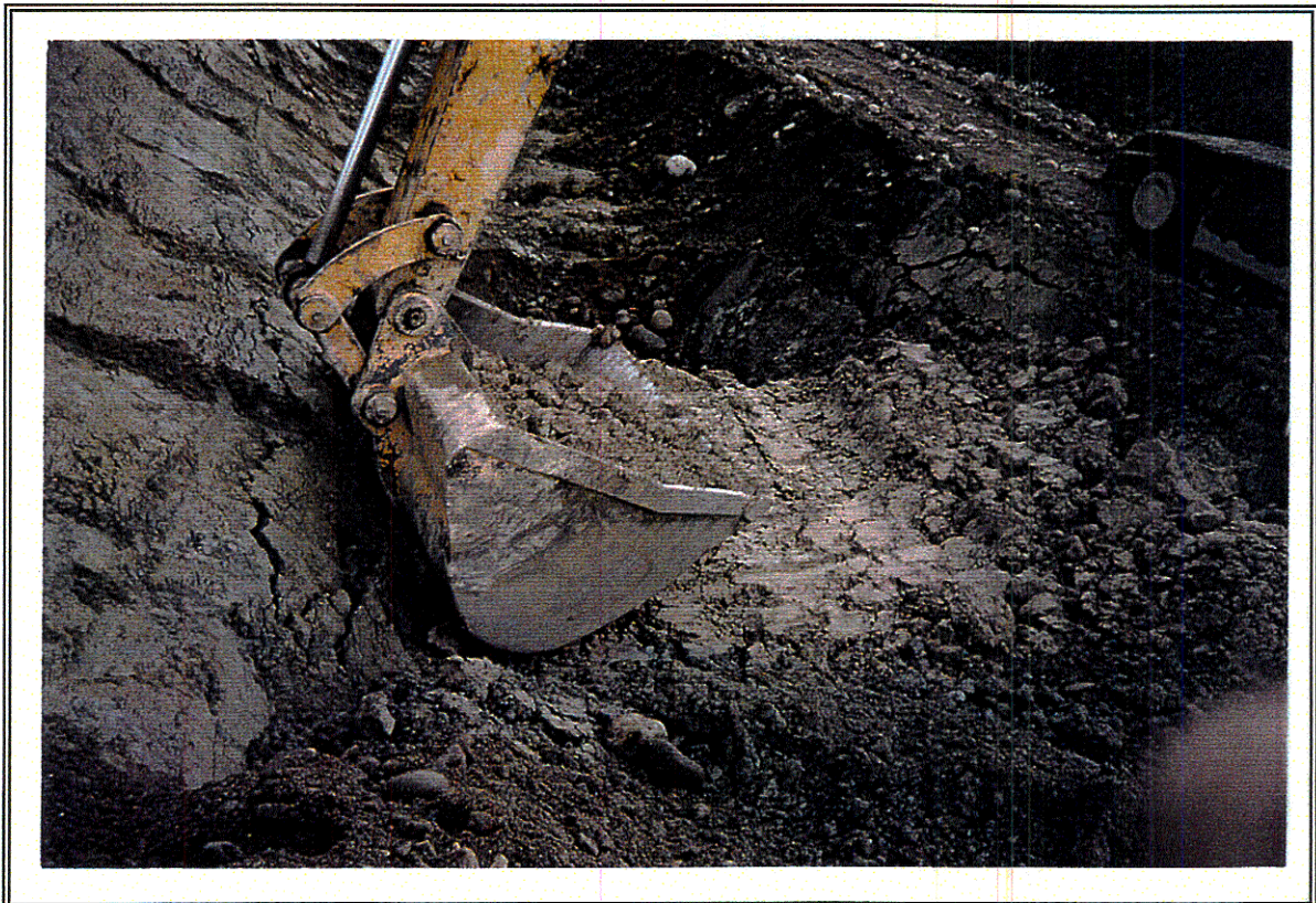
Figure 42: Hydraulic break construction.
