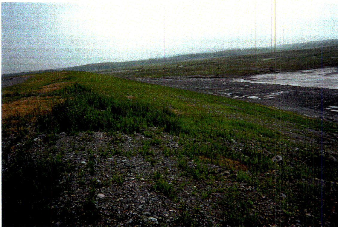
Photograph 2: South-East dyke after construction (fall 1998)
