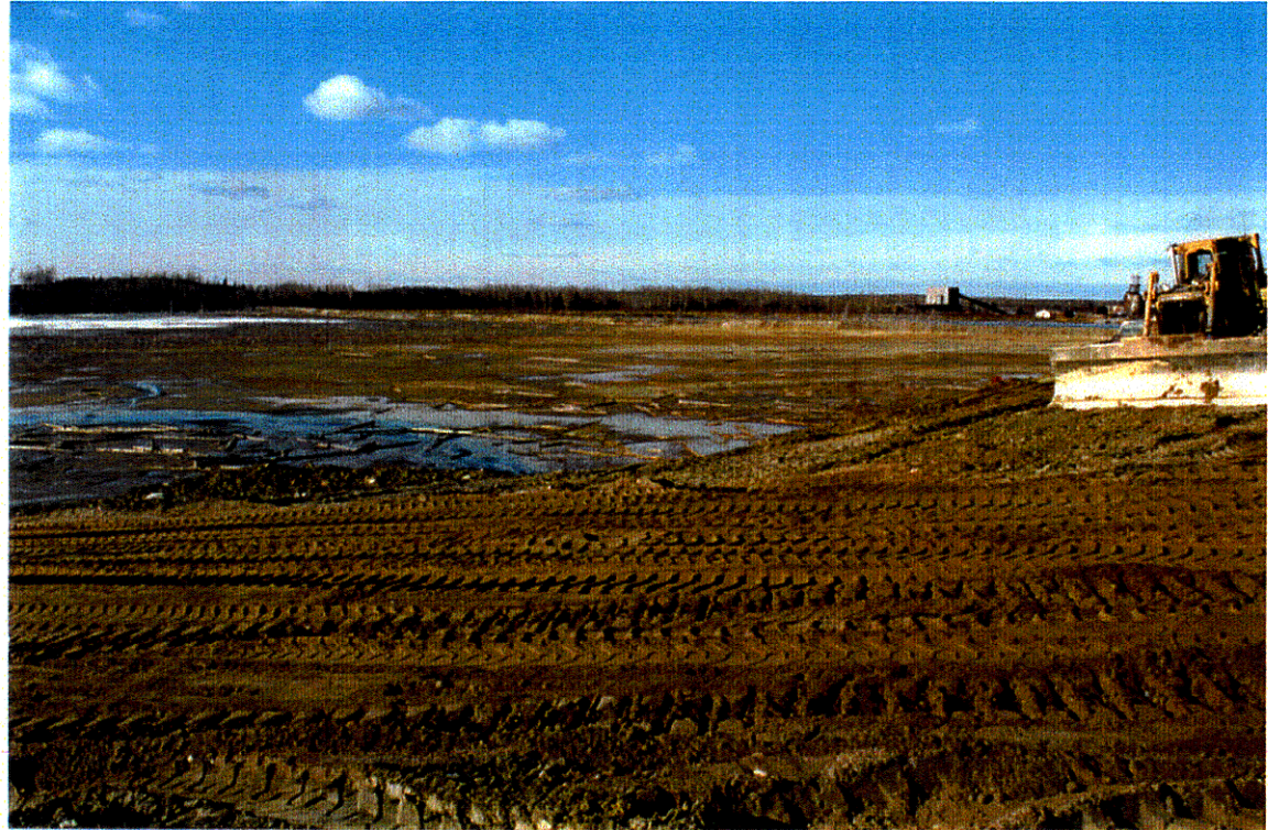
Photograph 3: West dyke before construction (fall 1995)
