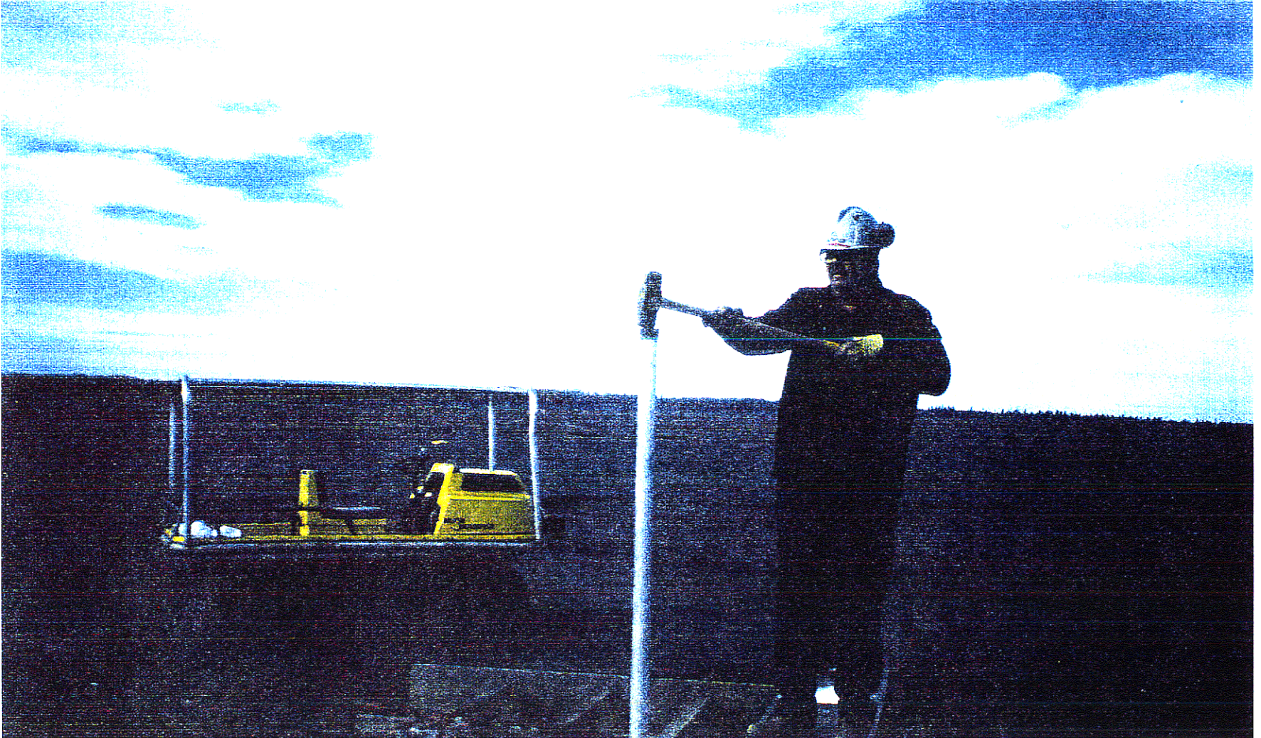
Photograph 4.2 INITIAL CORING SETUP
