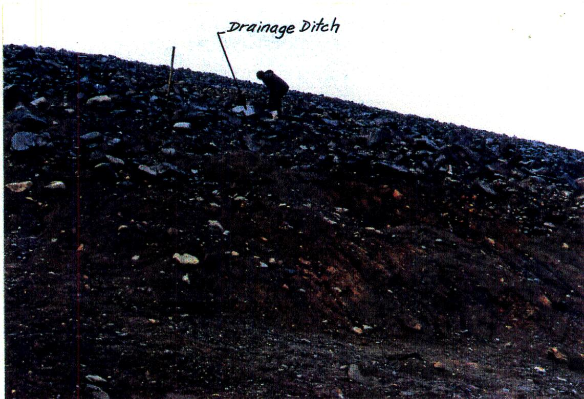
Plate 11: Killingdal - Covered rock pile showing location of drainage ditch
