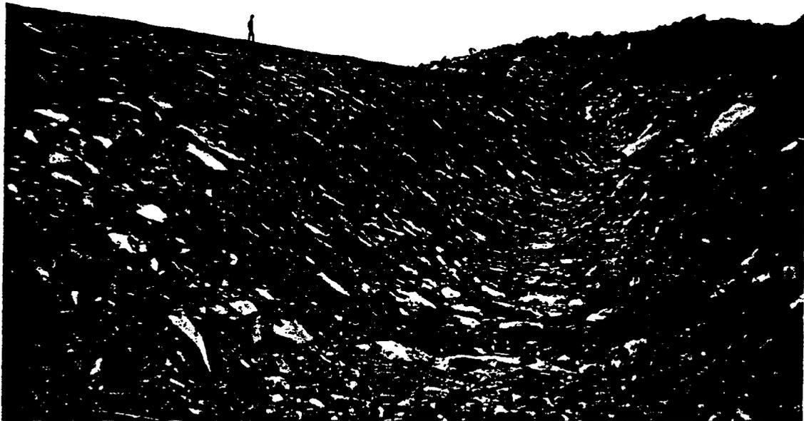
Plate 5: Kjølvi - Ditch at edge of rock pile into which geomembrane cover was sealed
