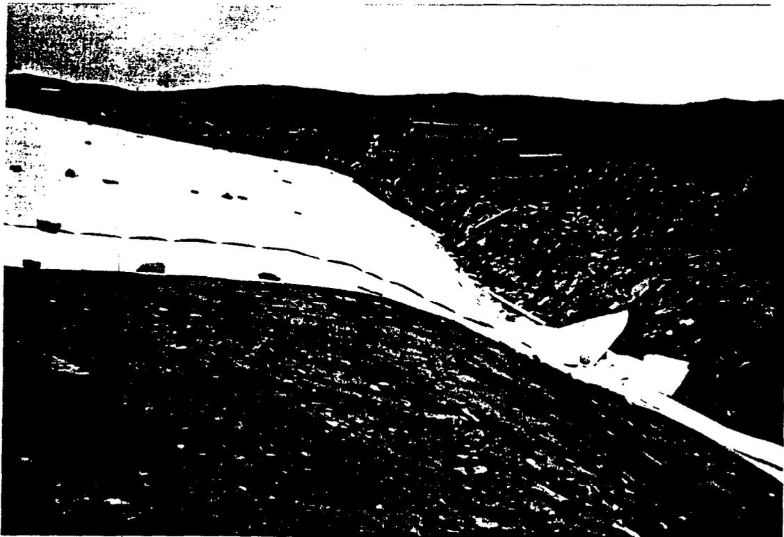
Plate 6: Kjølvi - Installation of lower geofabric layer and geomembrane
