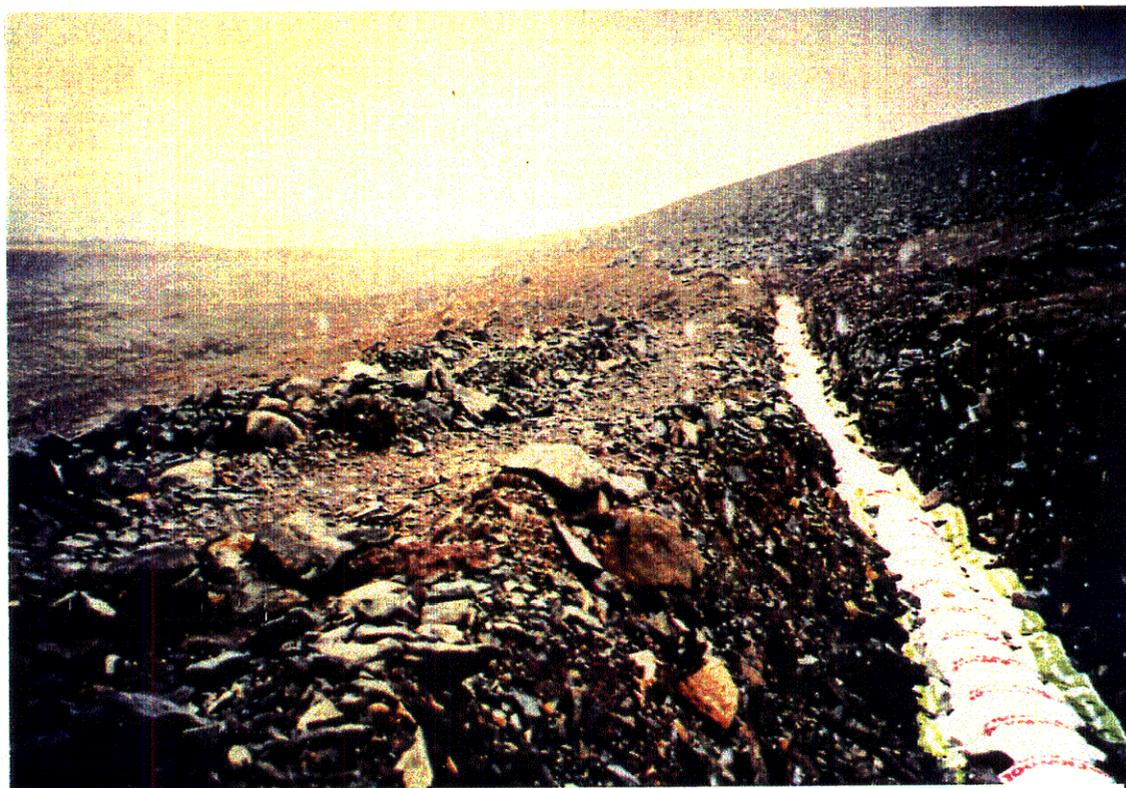
Plate 12: Killingdal - Portion of drainage ditch with drain pipes still to be completed
