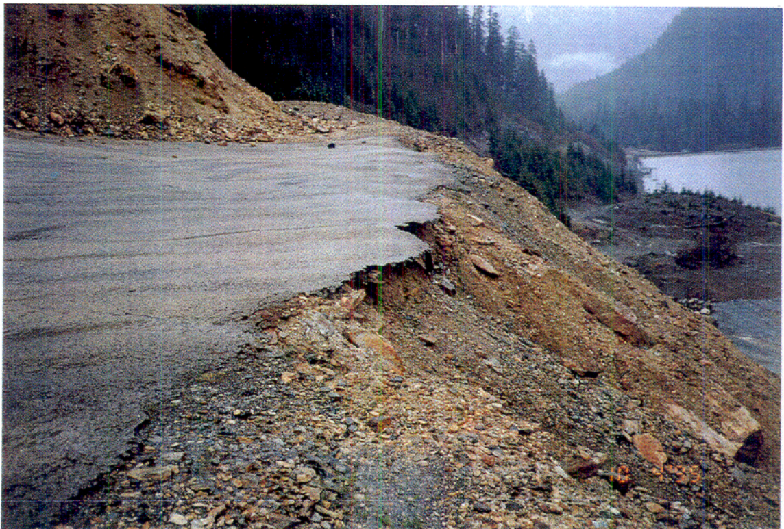
Photo 18 The edge of the lower portion of the test panel showed signs of erosion
