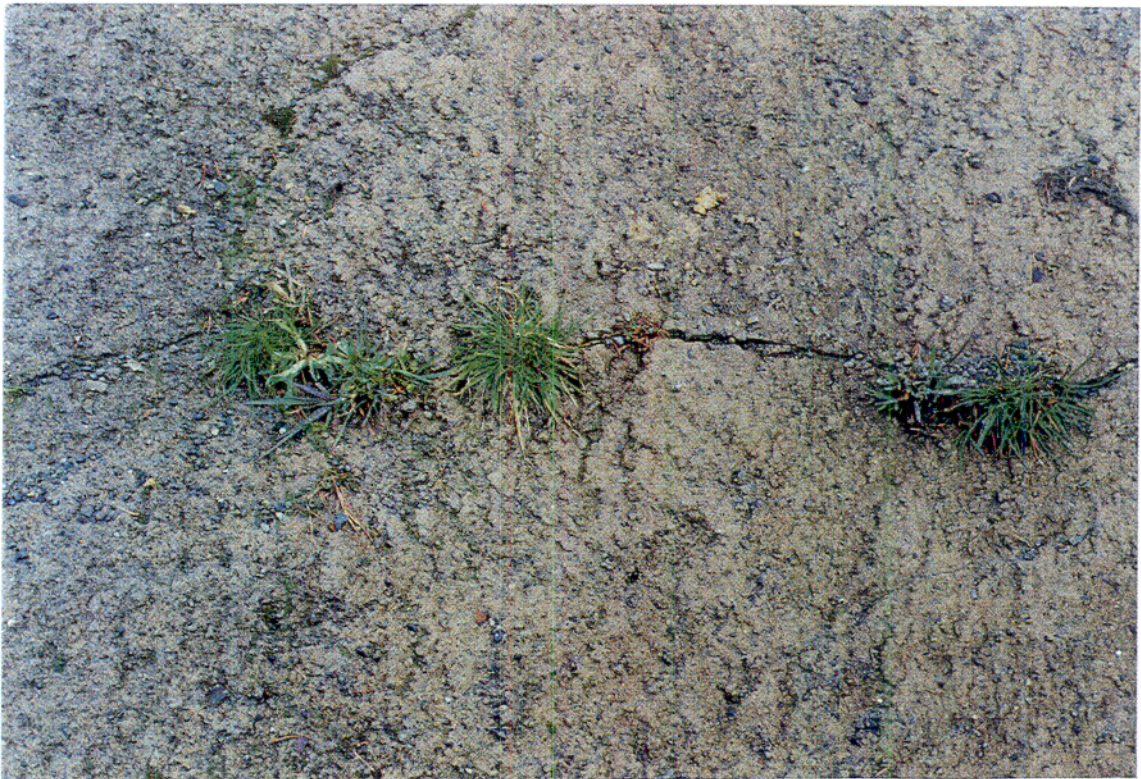
Photo 17 Vegetation and silt in few large cracks
