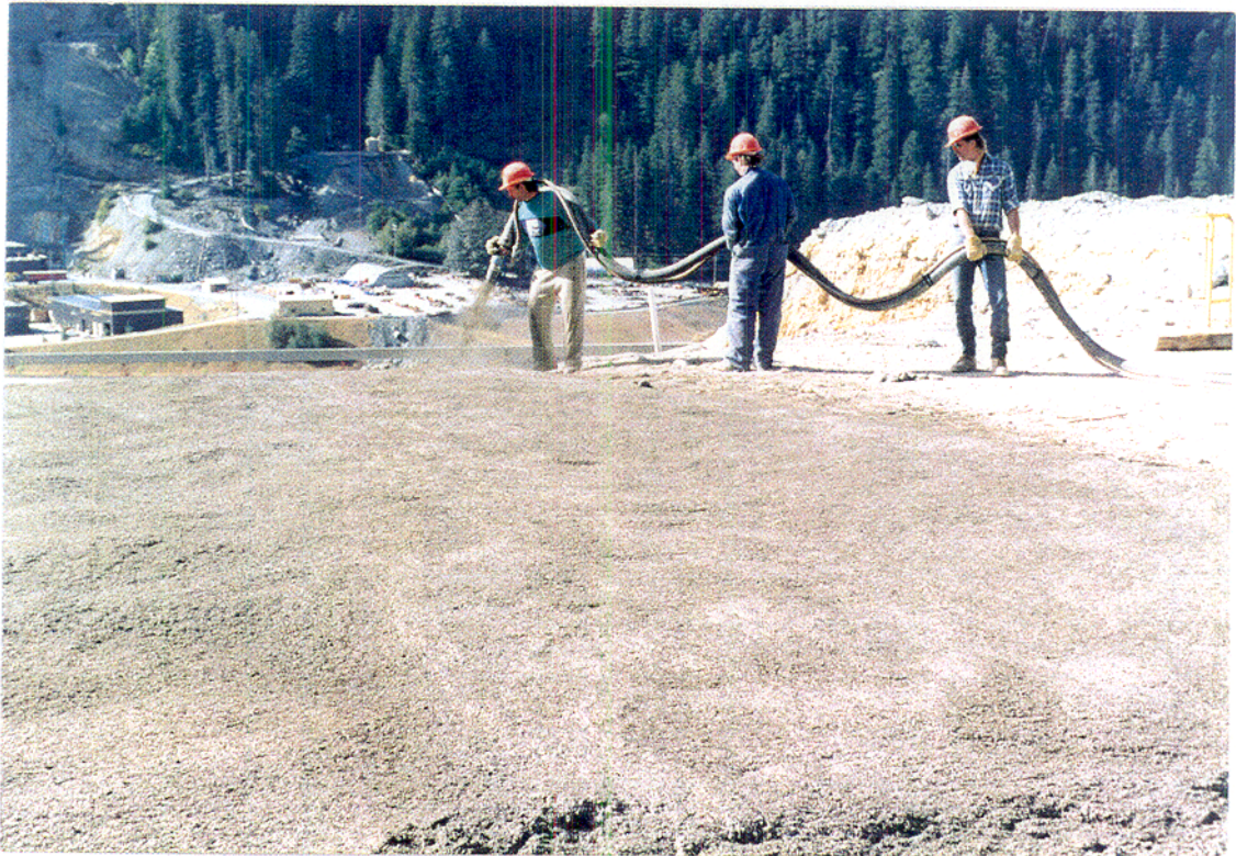
Photo 7 Nozzle was held manually where the robotic arm could not reach or when the robot was not working
