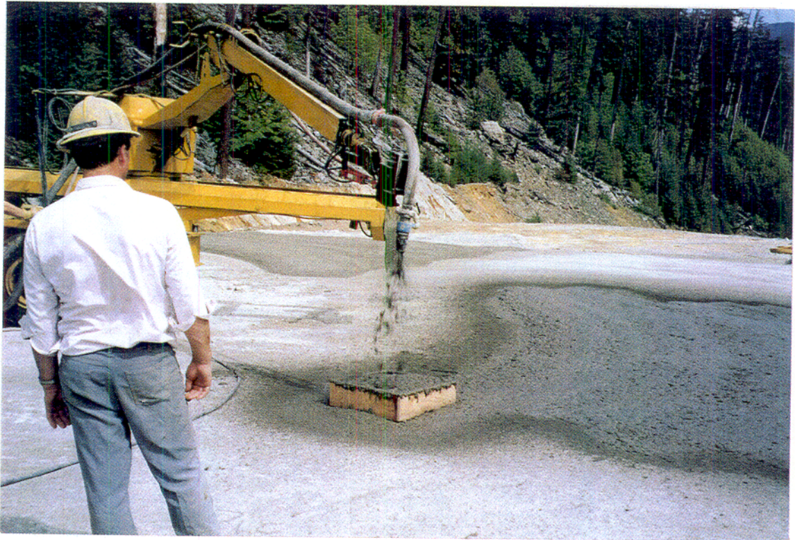
Photo 8 A panel was shotcreted for the laboratory test
