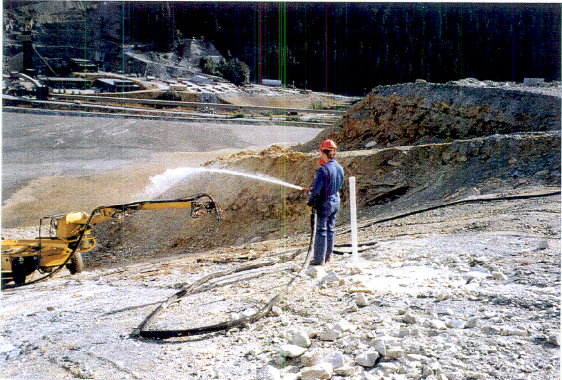
Photo 4 Water was sprayed on the waste dump before shotcreting
