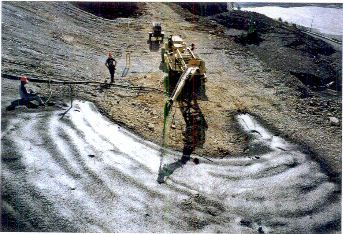
Photo 6 Robotic boom was swung side to side in sweeping motion and was slightly retracted after each sweep
