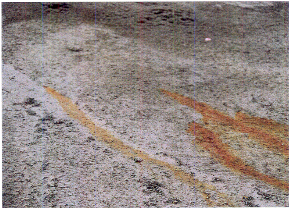
Photo 14 Oxide staining was observed on some areas as a result of water flow from the waste rock dump through the shotcrete panel
