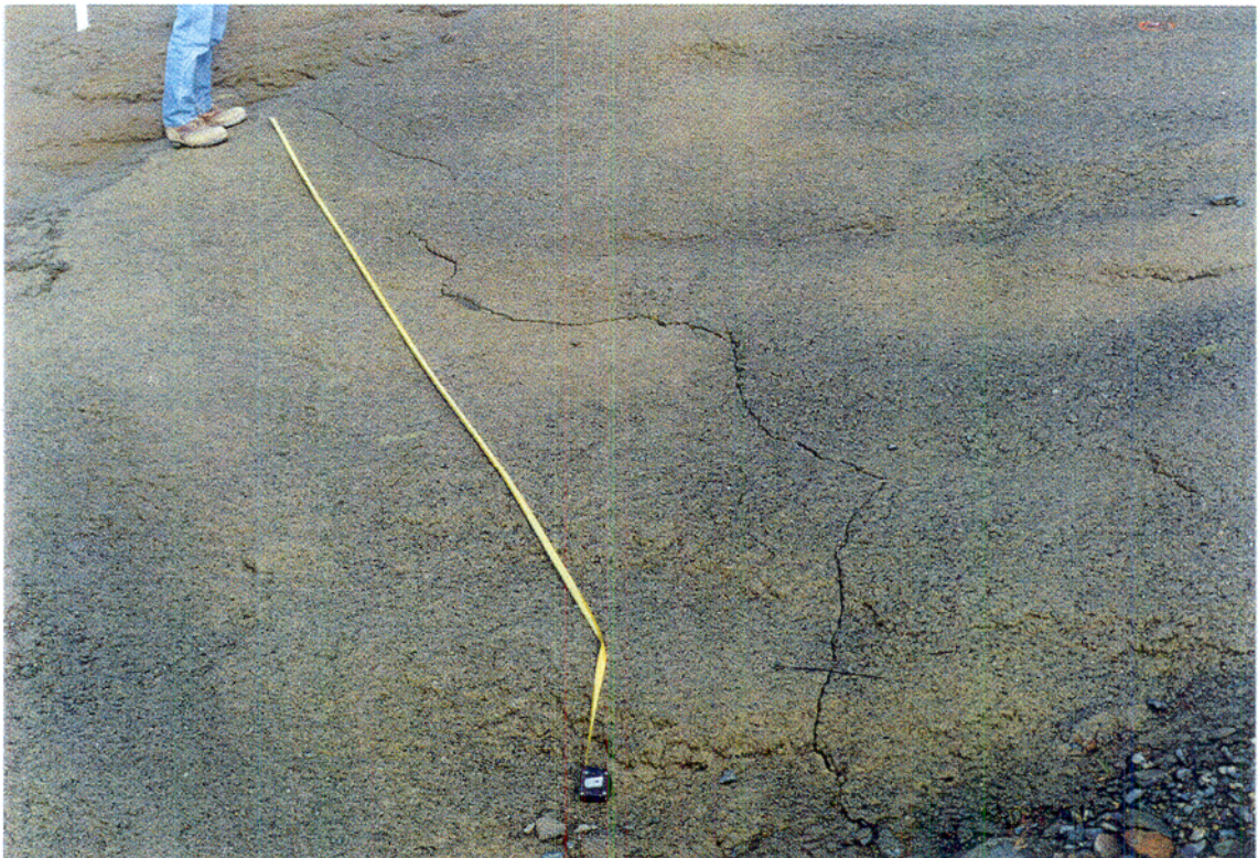
Photo 16 A 6m long crack located at between grid 37 and 54, as observed during 1995 inspection
