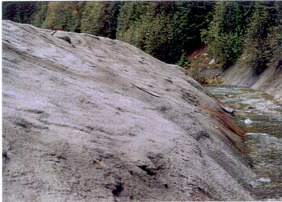
Photo 15 The shotcrete on the side of the diversion ditch as inspected in 1993
