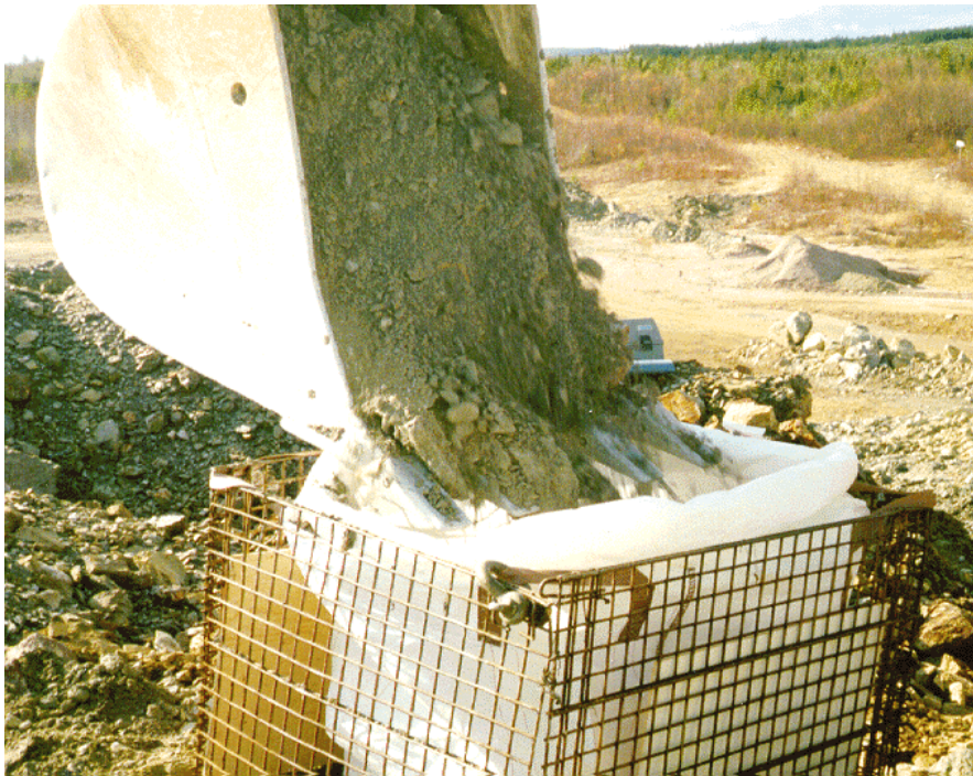
Figure 2-2 Bulk Sampling of Waste Rock on Stratmat Pile
