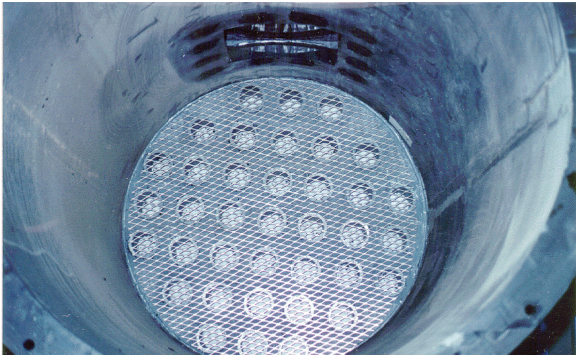
Figure 2-5 View of Installed Bottom Structure Looking Down Inside a Empty Column
