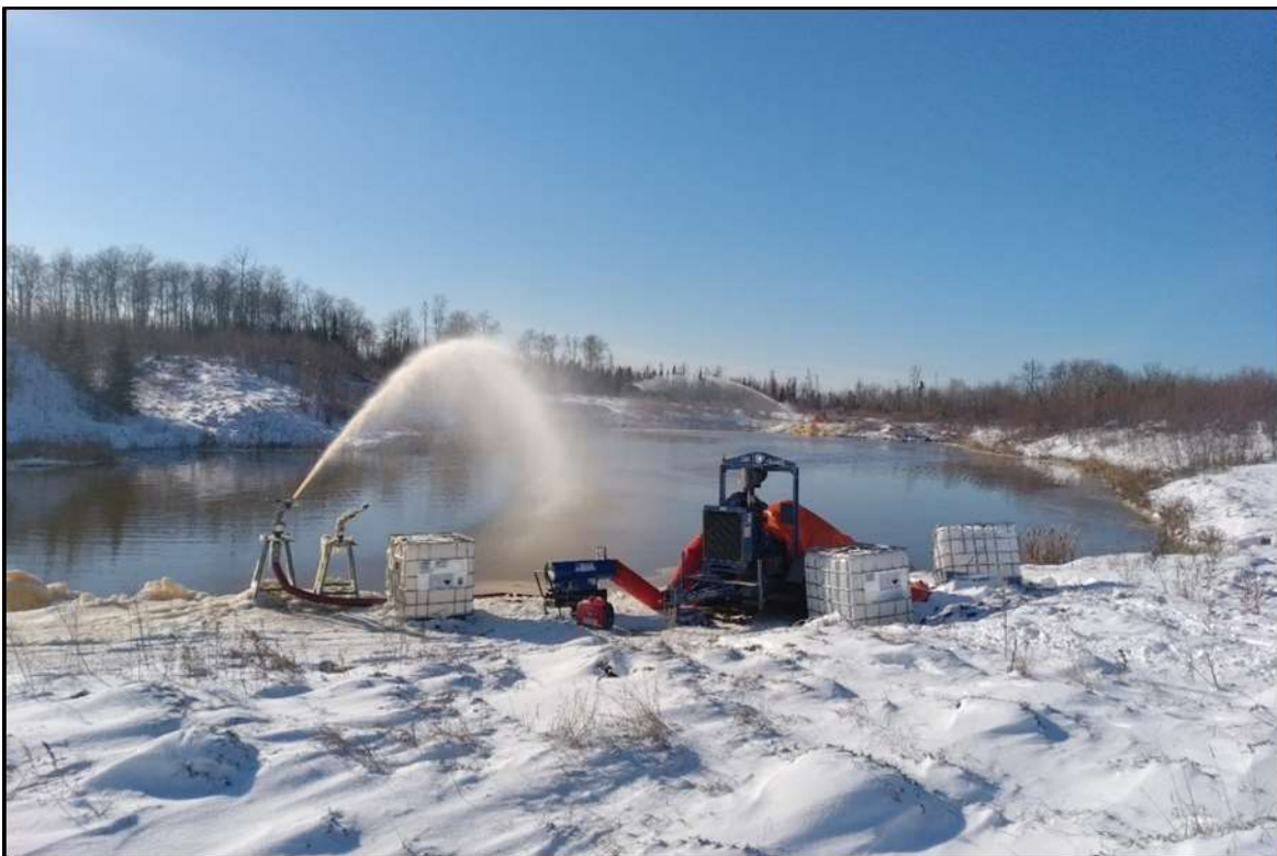
Figure 5-4: Near Completion of Application After Snowfall, Looking West.
