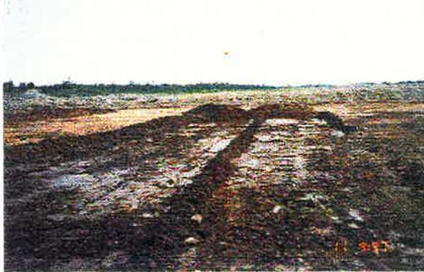
**Photo series G2. Dozing and backdragging (Cat D10N) in an area covered with about 10 cm of sludge deposited by dredge in 1994. 1995 July 11.**
