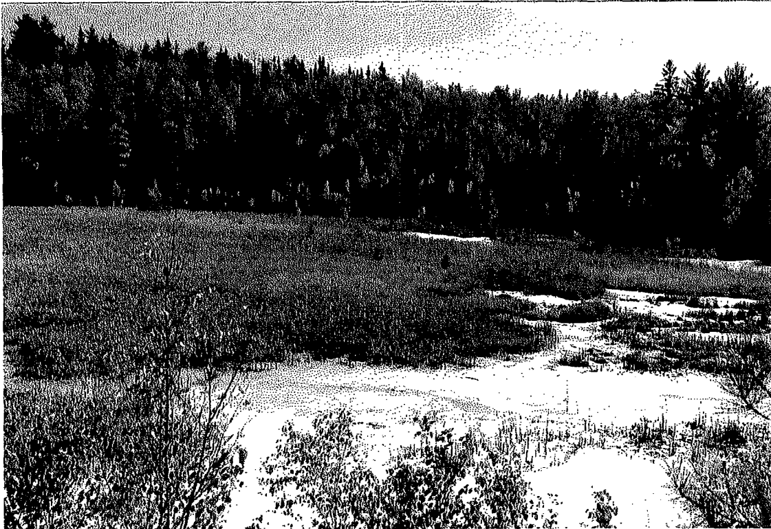
Fig. 6 - Oxidized and partially exposed tailings with vegetation, southwestern basin.
