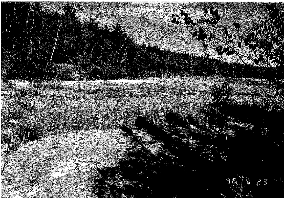
Fig. 4 - Oxidized and exposed surface of tailings with partially saturated and vegetation covered areas, western basin.
