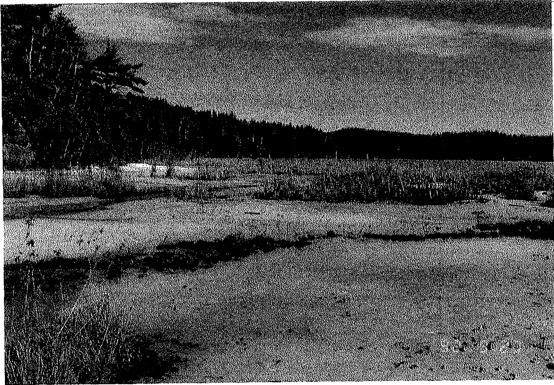
Fig. 5 - Oxidized and exposed surface of tailings with partially saturated and vegetated areas, northwest part of the basin.
