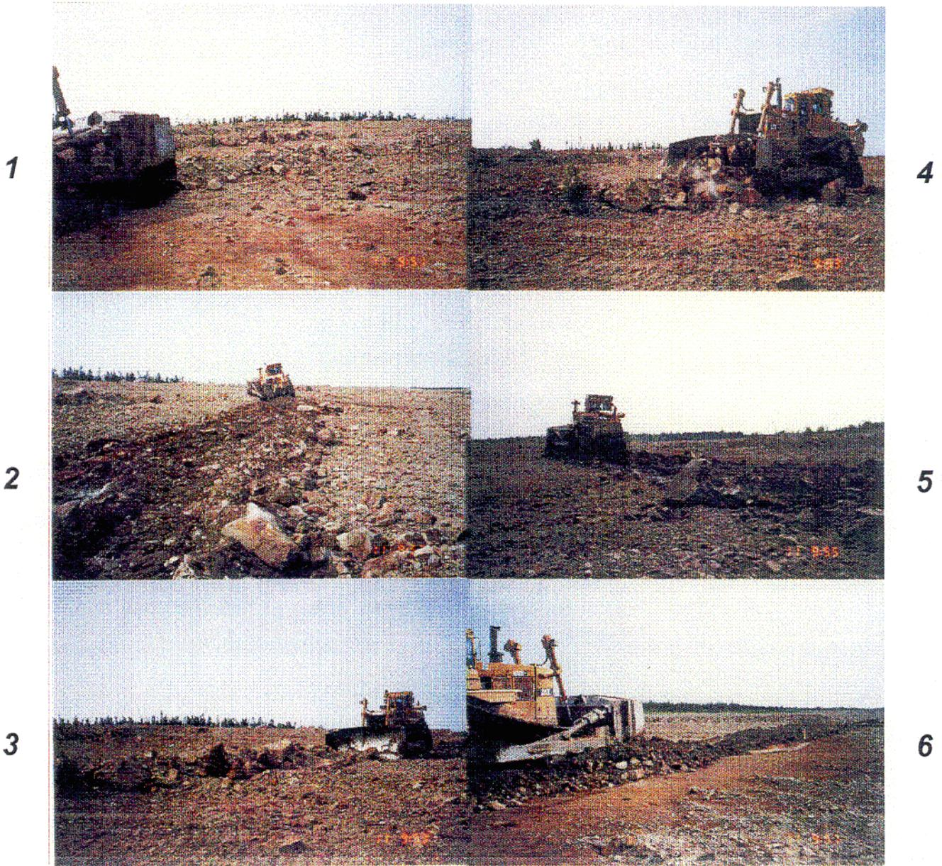
***Photo series G5. Transforming an extremely rocky area to a relatively even surface by burying, crushing or removing the larger-size rocks (Caterpillar D10N). 1995 July 11.***
