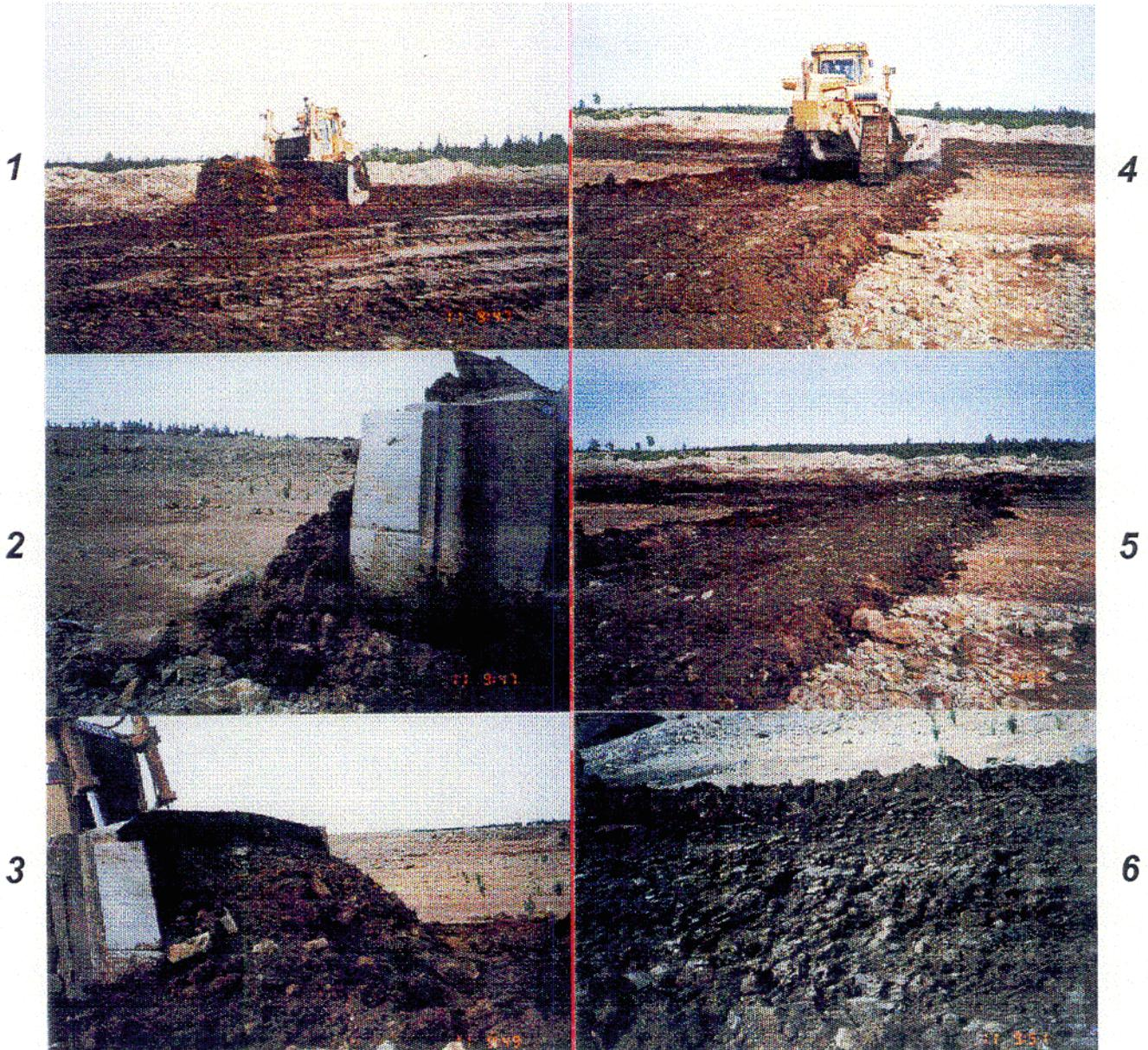
**Photo series G4. Mixing of piled-up and pumped sludge (G4-1) with near-surface rockfill (Caterpillar D10N). 1995 July 11.**
