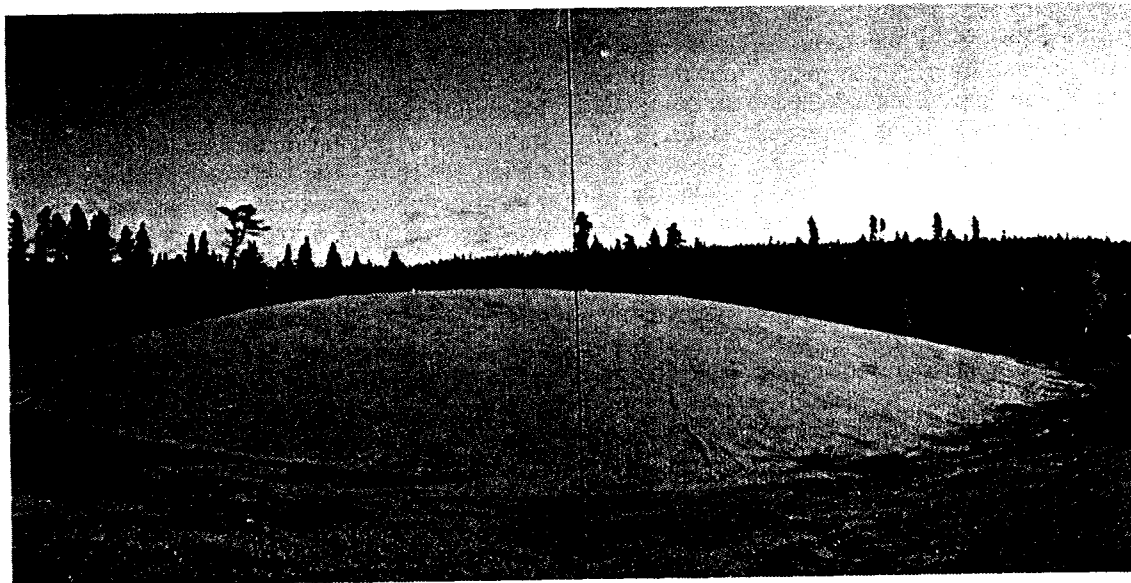
FIG. 8. Waste rock pile 7/12 after cover installation.
