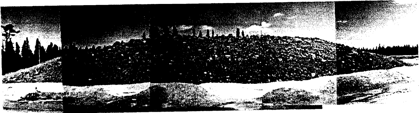
FIG. 7. Waste rock pile 7/12 before cover installation.
