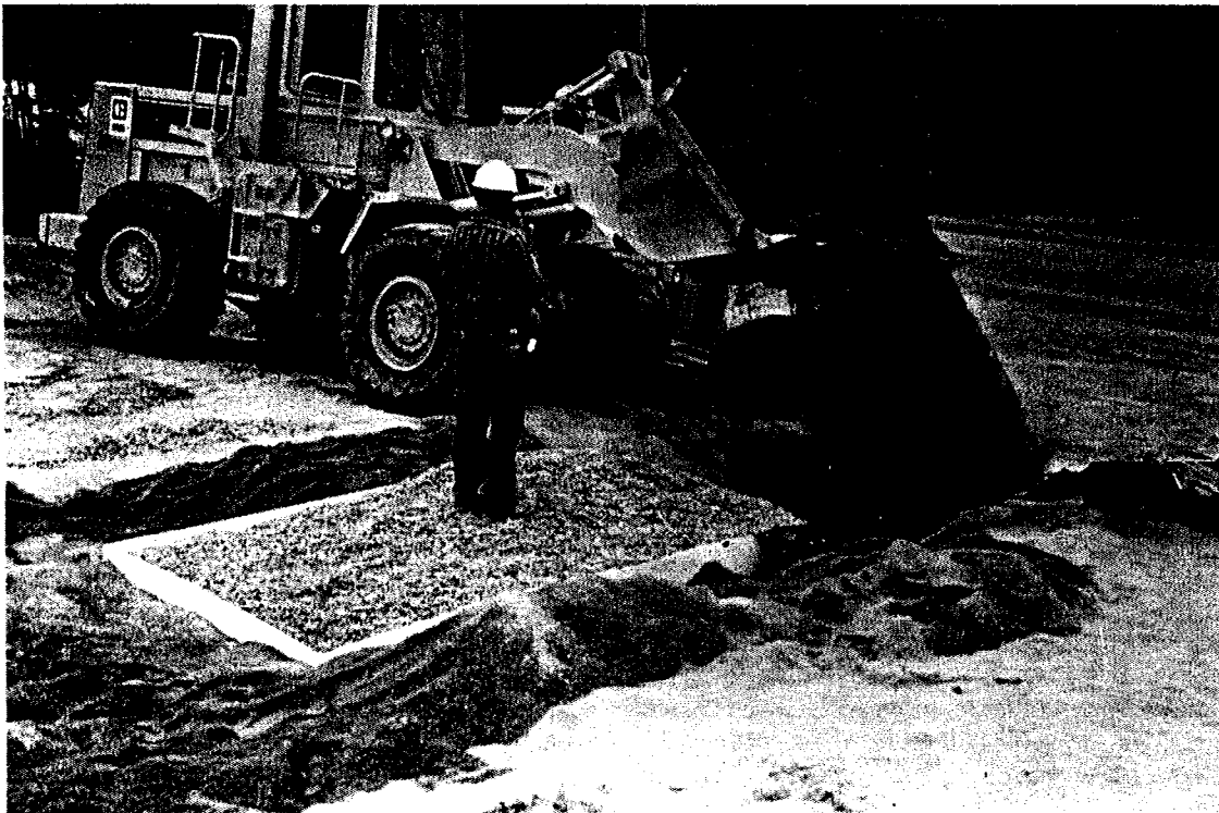
FIG. 10. Backfilling of northeast lysimeters following installation.
