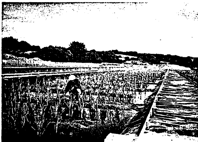
The pilot-scale passive-treatment system at the Wheal Jane Mine in Cornwall, England is designed to treat 42 L/sec (665 gpm) of ARD (pH 3.0, 250 mg/L iron, 250 mg/L zinc).
