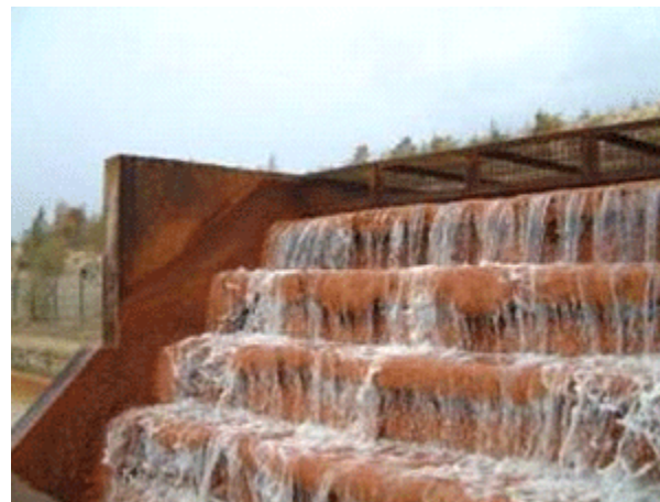
Figure 8-20: Aeration Cascade for Oxidation of Coal Effluent (88)
