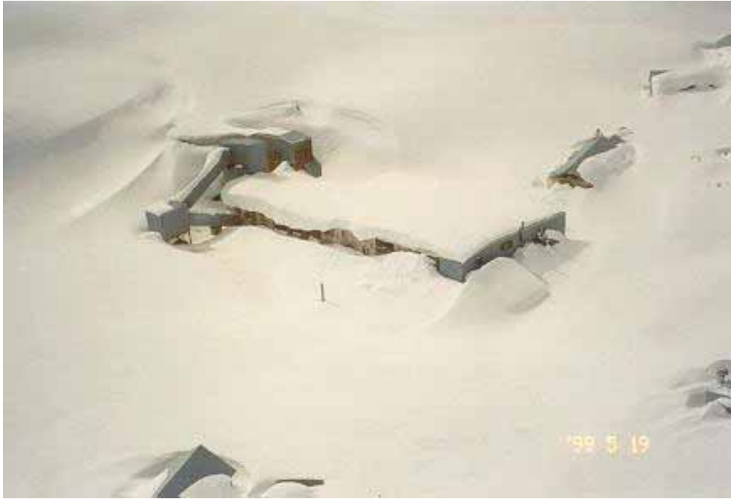
Photo 5. The Camp and Plant Site on May 19th, 1999
